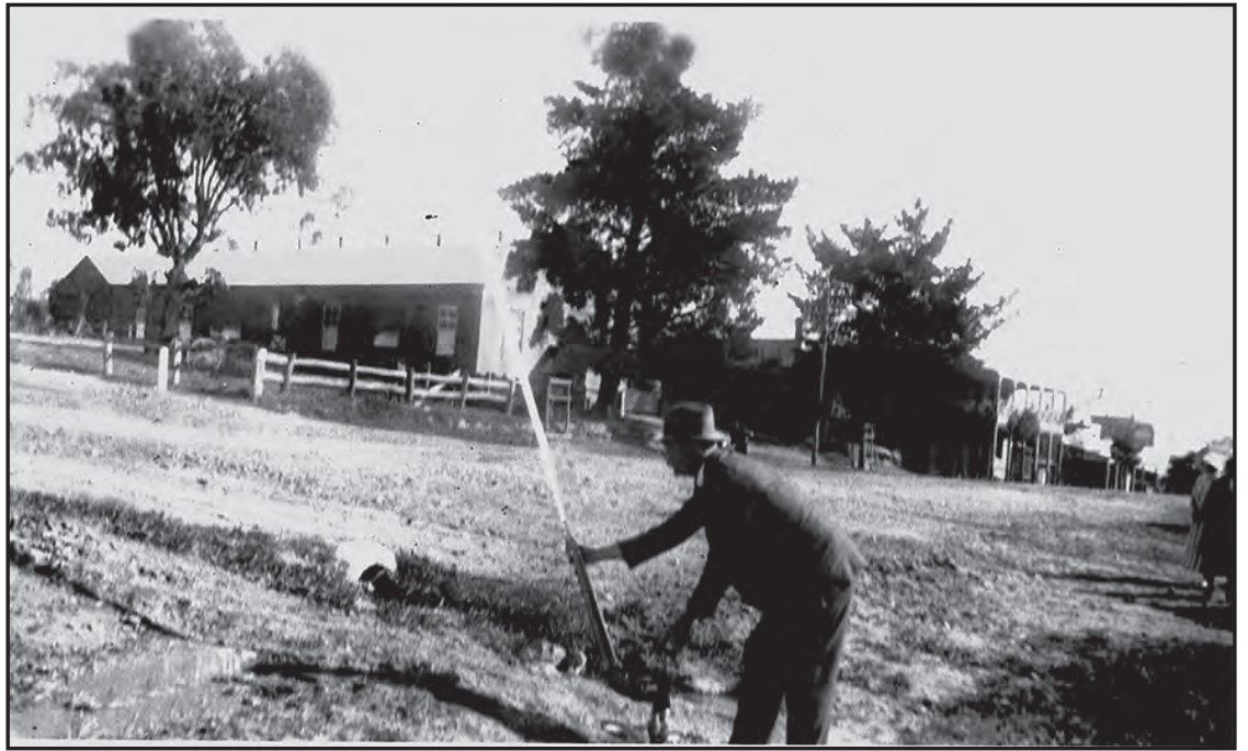
Local Water Commissioner, Alfred Acocks, turning the tap to release the first water from Corryong's newly-constructed reticulation system in 1924.
