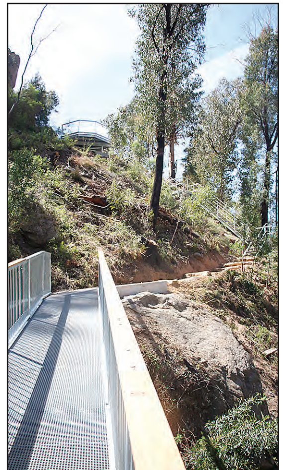
A fire-resistant stairway leads to the main viewing platform.
