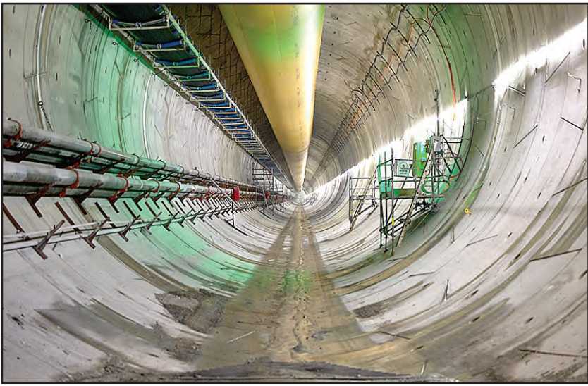
The tailrace tunnel will link with the new power station.
