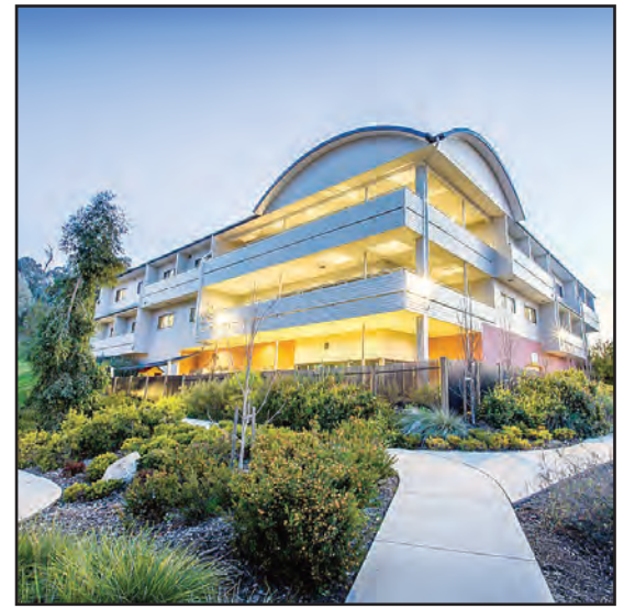
The first stage of the accommodation centre has been completed.
