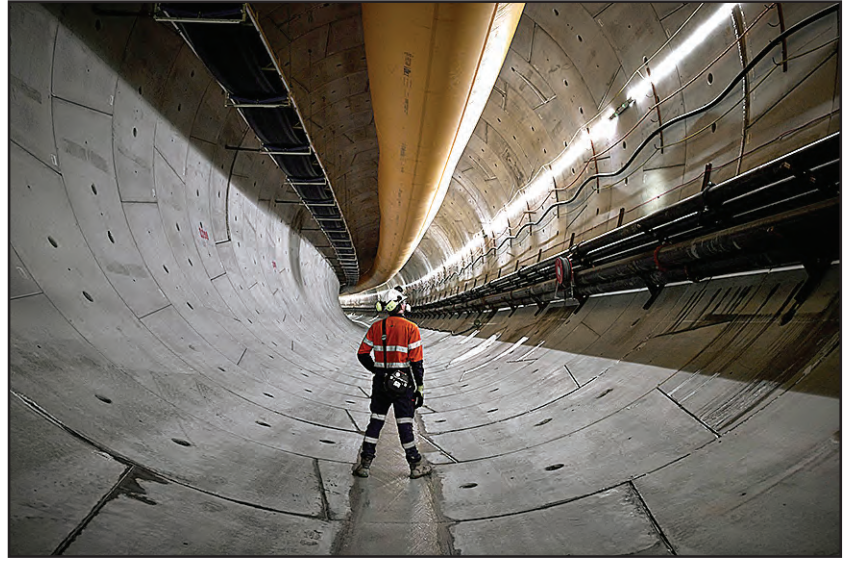
The main access tunnel has been completed.
