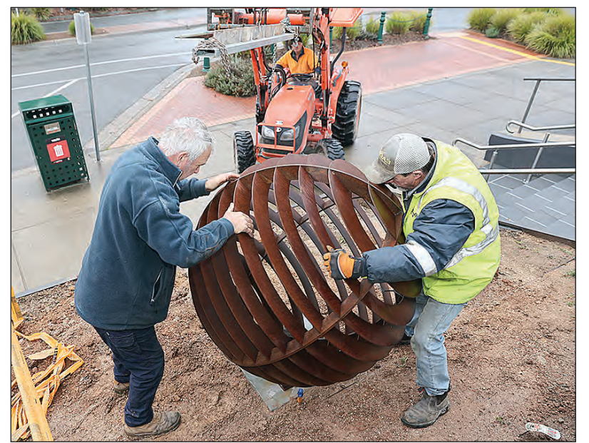
Local electrical contractor, John Collins (left) installed a new feature light at the Corryong Memorial Hall this week with the assistance of Gary Barker (right) and Ross Collins.
