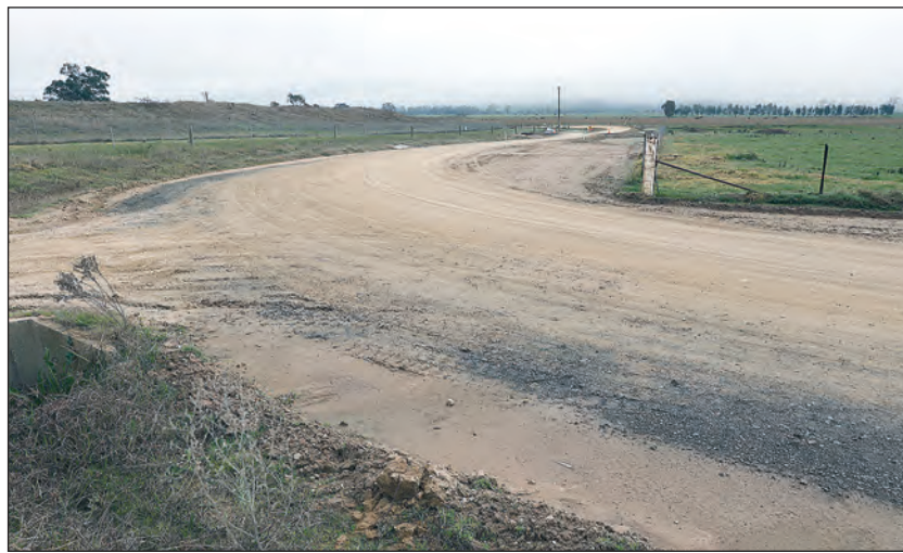
Tight corners are being removed along the new route.
