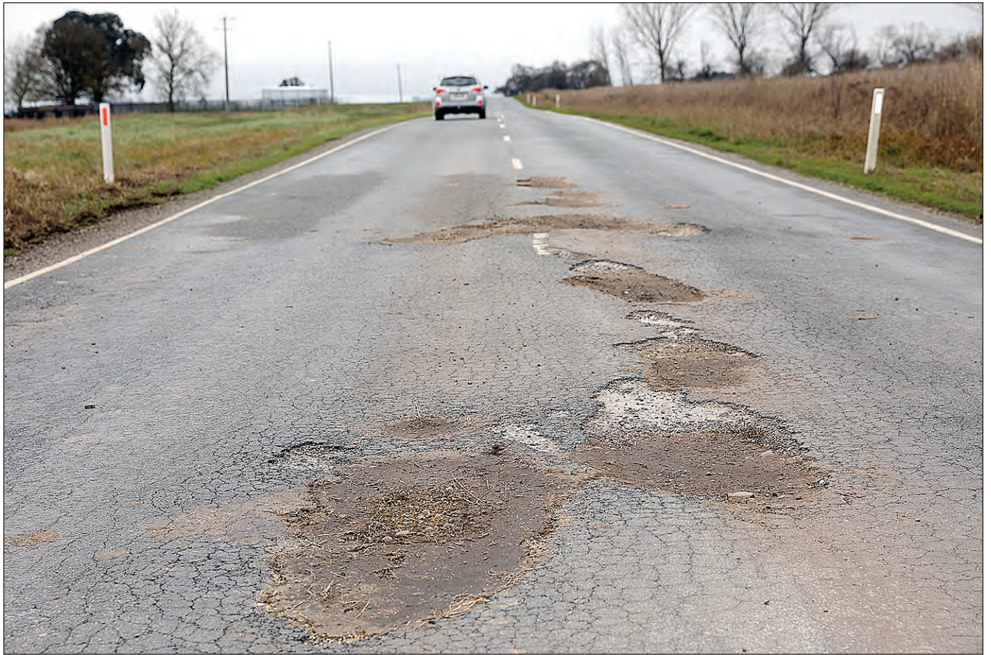
This section of the Murray Valley Highway between Corryong and Towong was repaired earlier in the year but recent wet weather has caused even more extensive damage to the roadway. Its condition could have been worse if not for a couple of civic-minded locals who have taken it upon themselves to fill in potholes in Corryong and surrounds.
