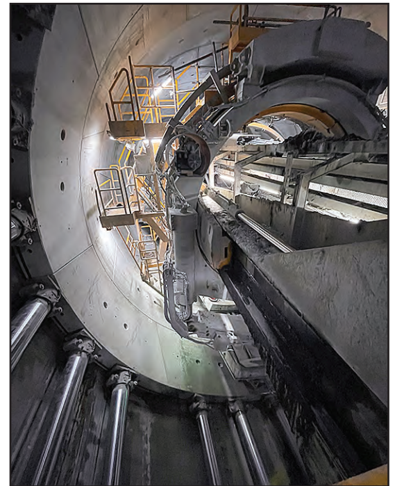
The first Snowy 2.0 tunnel was completed in October last year.
