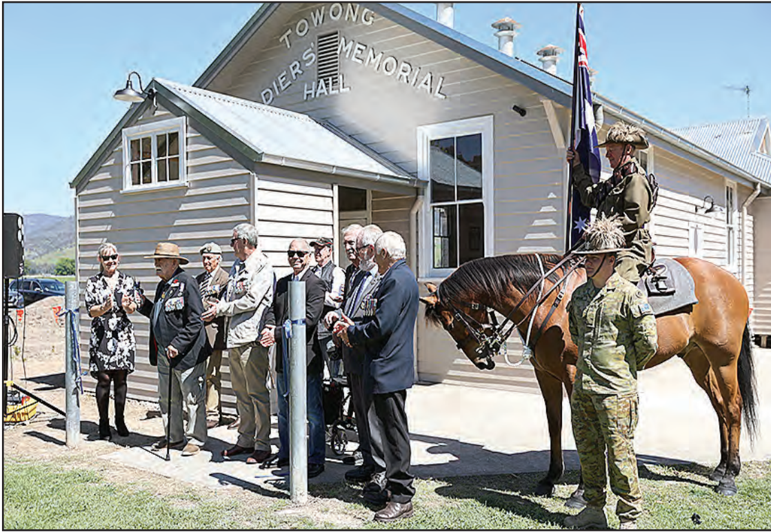
The Towong Hall renovation was the latest recovery project to be completed.
