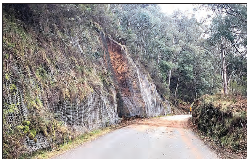
Slope strengthening work may cause traffic delays.
