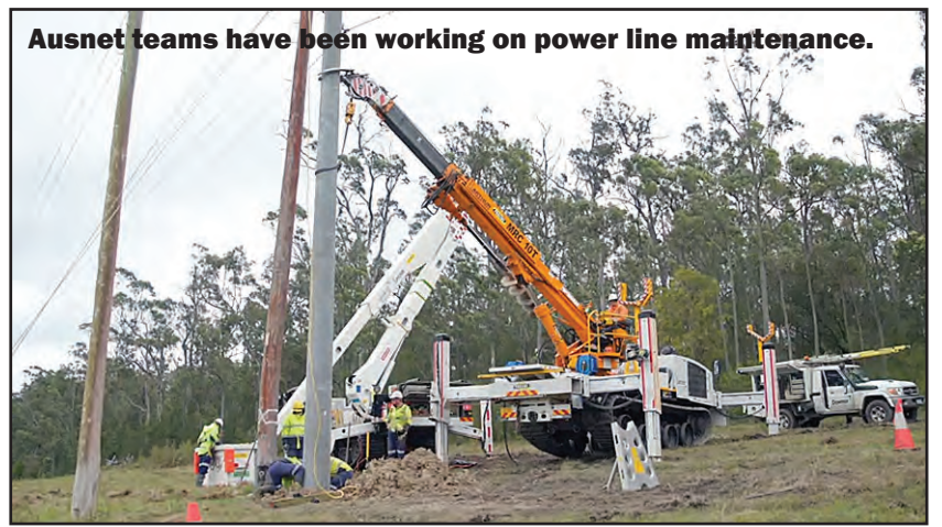
Ausnet teams have been working on power line maintenance.
