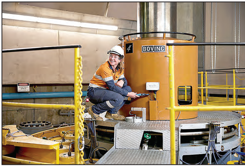
Sallie Findlay works on a turbine at Murray 1 power station.
