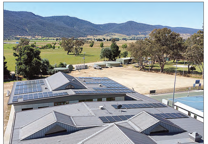
A community energy system at the Corryong Events Centre is nearing completion.
